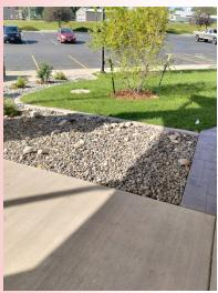
As a result of the extensive grading and excavation, the majority of the existing landscaping was removed. Decorative concrete aprons were installed adjacent to the building to
